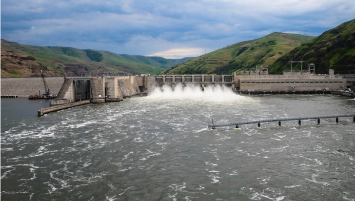
Lower Granite Lock and Dam
